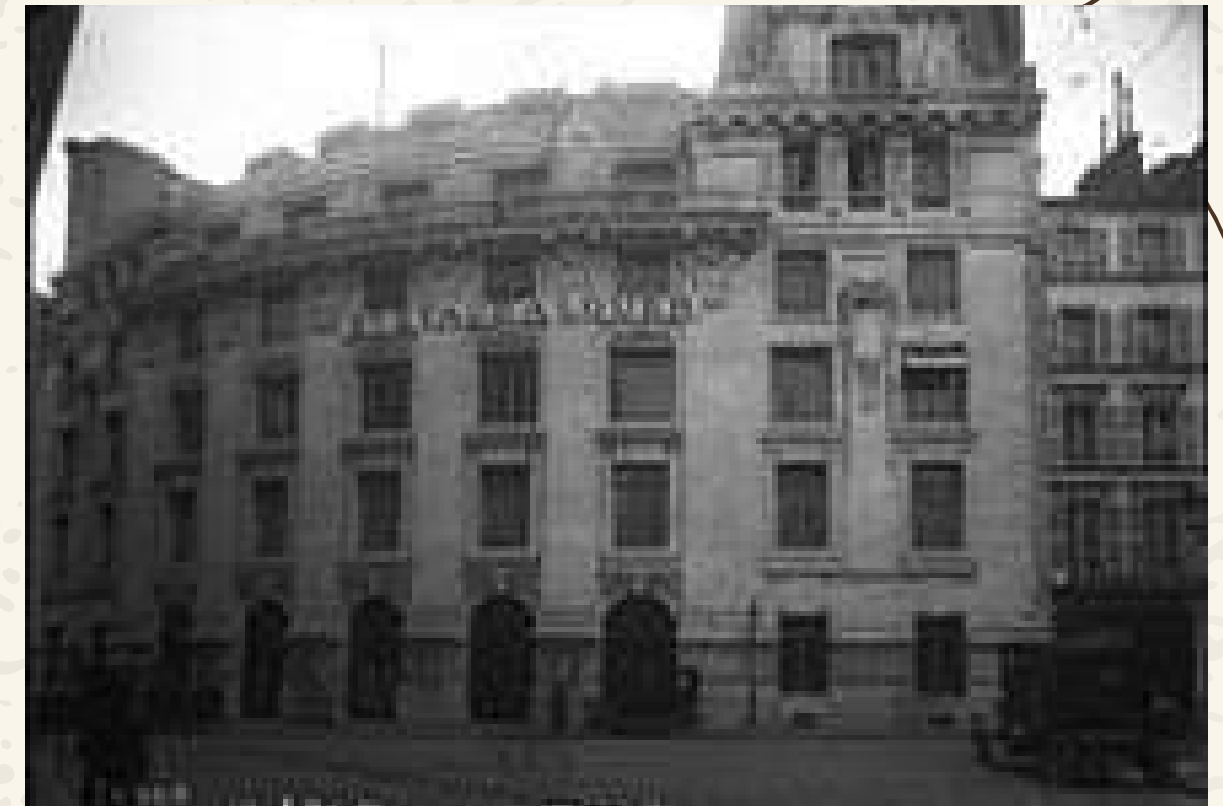
Headquarters of Crédit Mobilier
